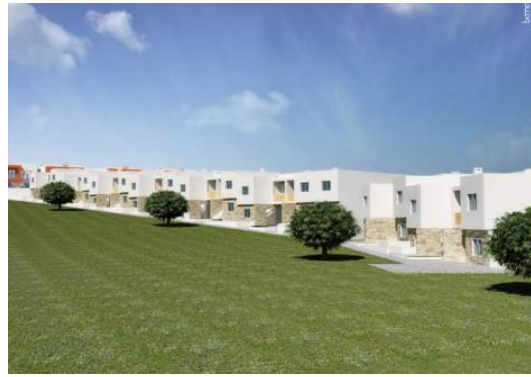
Gated condominium under construction
