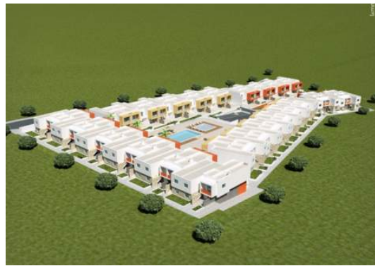
Gated condominium under construction
