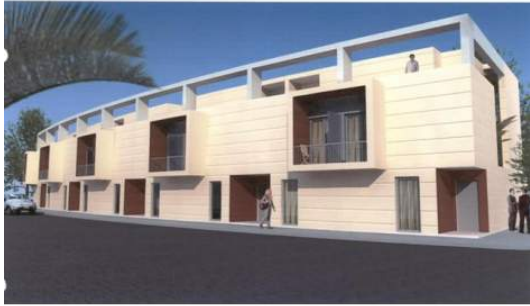
3 Bedroom townhouses under construction
