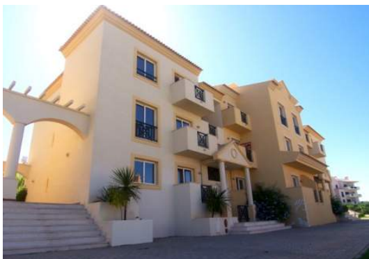
Front of building
